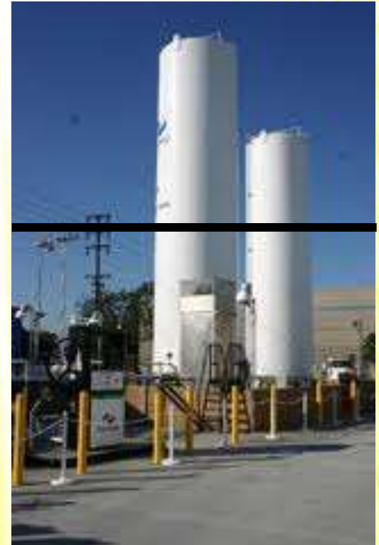
Boil-off 0,1%/day, after 10 days, storage half empty. 375 liters of methane lost. Composition of remaining LNG increased in C2/C3
