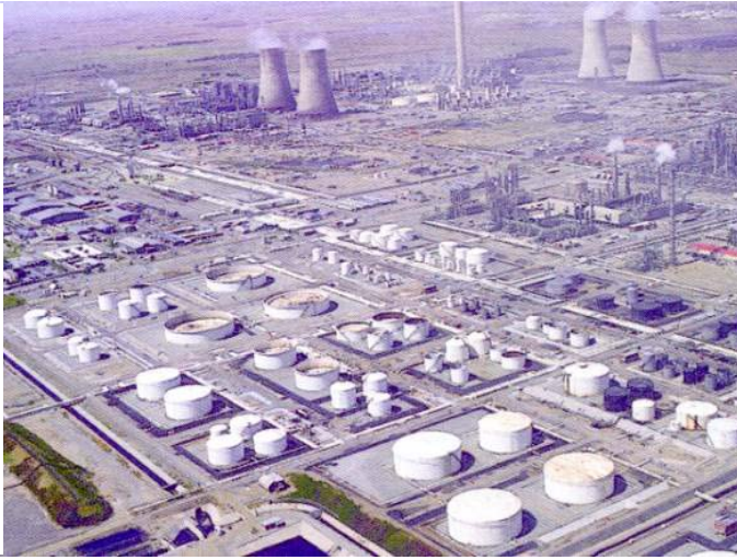
Largest O2 site in the world 42 000 mTPD - SASOL
