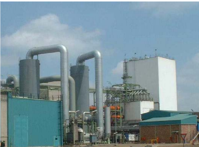
Largest ASU trains in the world 4 200 TPD (at MSL) - SASOL T15
